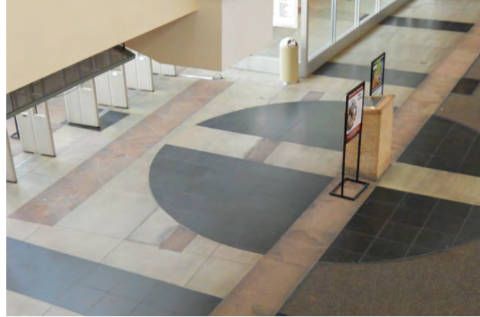
the existing entry foyer and lobby has a monolithic slab with a variety of stone insets creating a prominent design at the entry of the building, this area could remain as it is not the problem area
