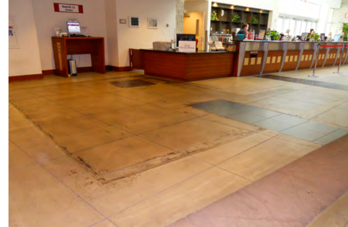
circulation desk area showing the glue marks and discoloration from the carpet inserts that were removed
